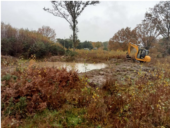
Pond work on Pound Common
