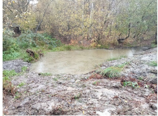
Pond clearance on Memorial Common
